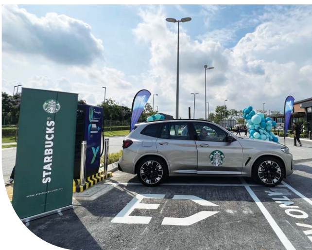
EV charging machines in BStarbucks Drive-Thru stores.
