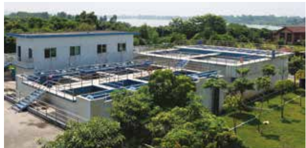
The Pengfa water treatment plant in China.
