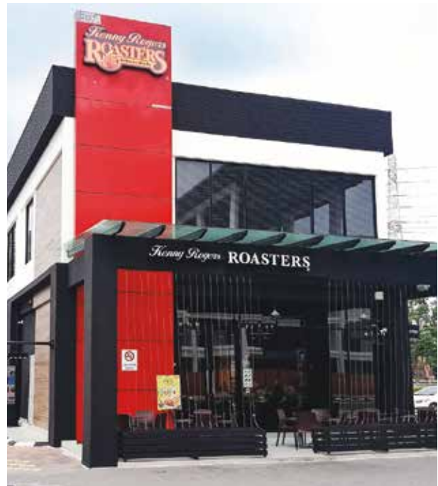
KRR Drive-Thru outlet in Juru, Penang.
