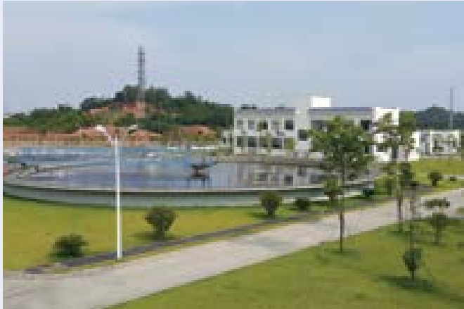
The Jinben wastewater treatment plant in Sanshui District, Guangdong Province, PRC.
