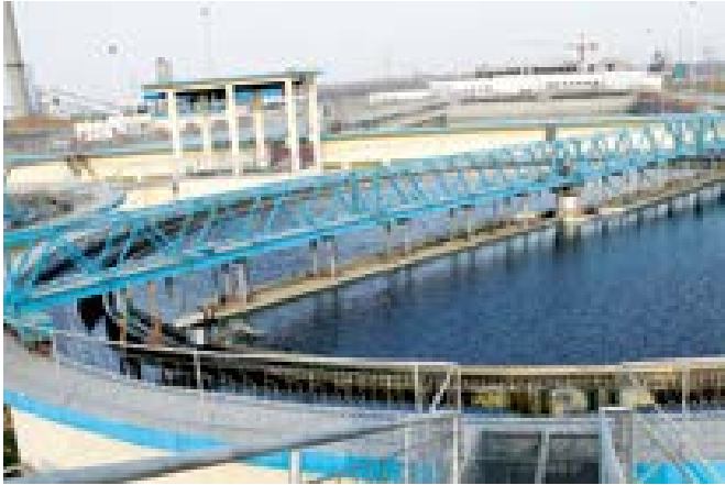
Secondary Sedimentation Tank of DSG's Taian Sewage Treatment Plant in the PRC.
