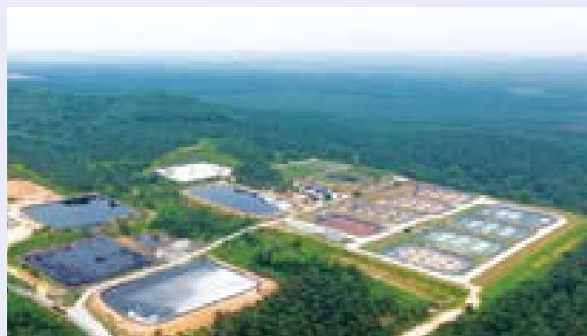
Aerial view of the Leachate Treatment Plant at the Bukit Tagar Sanitary Landfill, Selangor.
