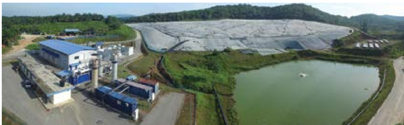
The Renewable Energy Center at the Bukit Tagar Sanitary Landfill, Selangor.
