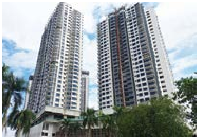
Construction is in progress for The Link 2 @ Bukit Jalil, Kuala Lumpur.
