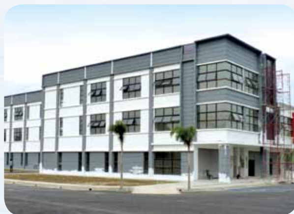
Completed Phase I of Trade Point, Berjaya Park, Shah Alam, Selangor.
