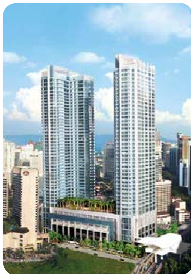
Menara Bangkok Bank @ Berjaya Central Park, Kuala Lumpur.
