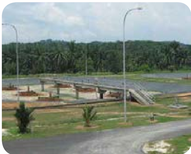
Leachate treatment plant, Bukit Tagar Sanitary Landfill, Selangor.
